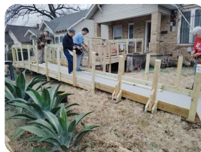
Ramp for Wilma Smith on N. 12th St
