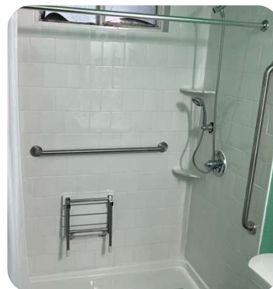
Accessibility installations for the Lawrence Family on Avendale
